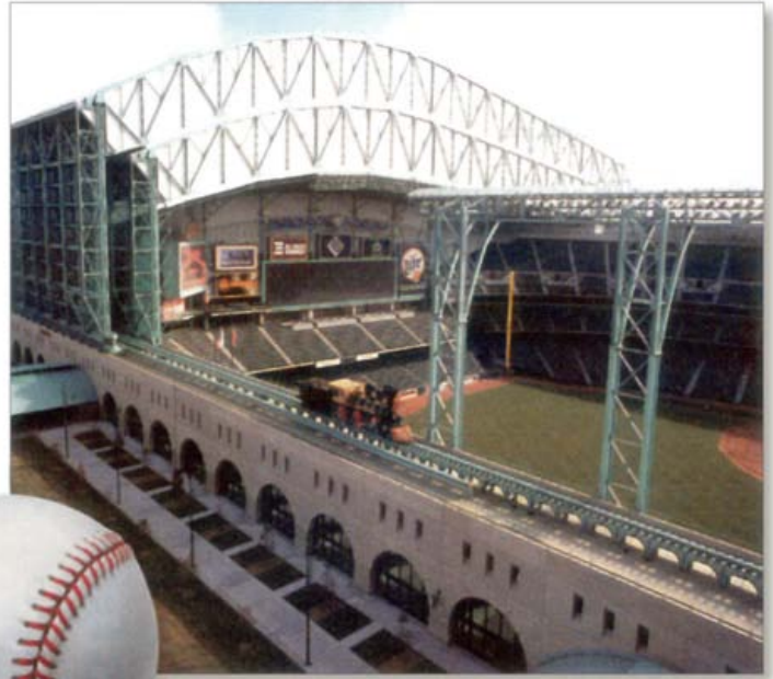
The retractable roof at Houston's Enron Field rides on suspension springs made of Adiprene urethane.
